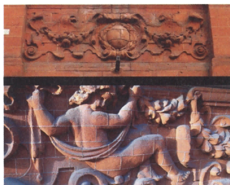
Top Facade and brickwork details.
