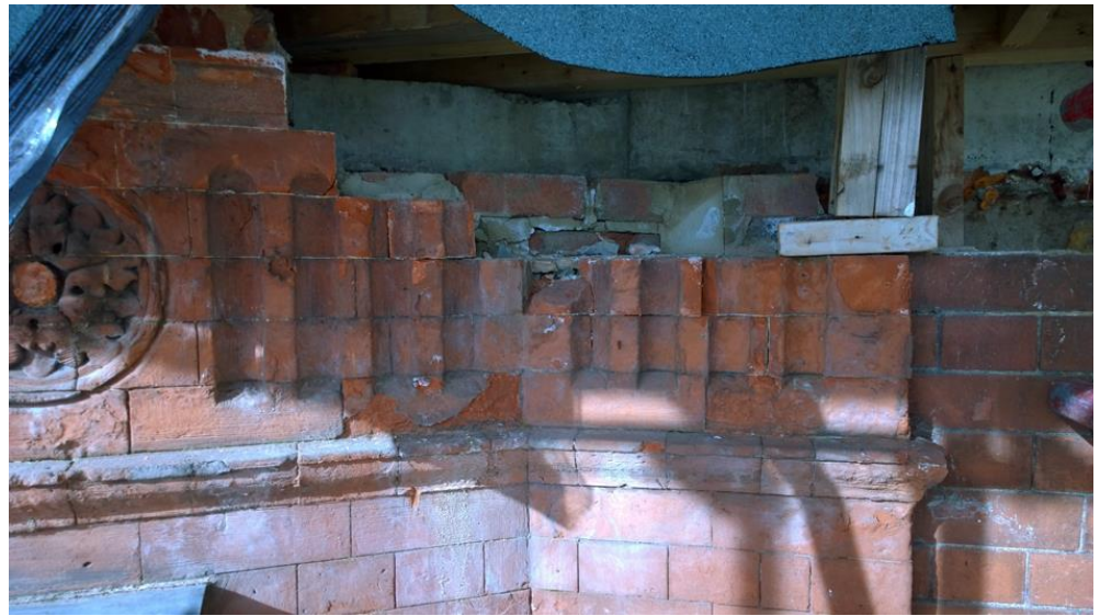
Building no.1 - Retained Façade Failure: Spalling (water ingress)
