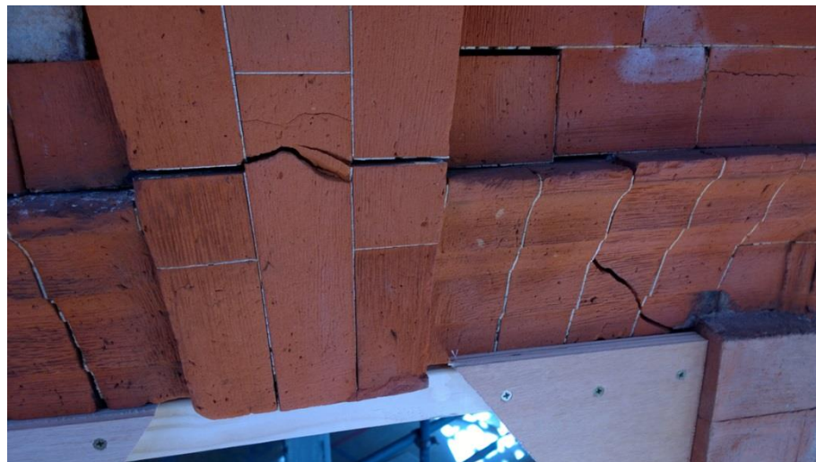
Building no.1 - Retained Façade Failure: Slippage + Movement
