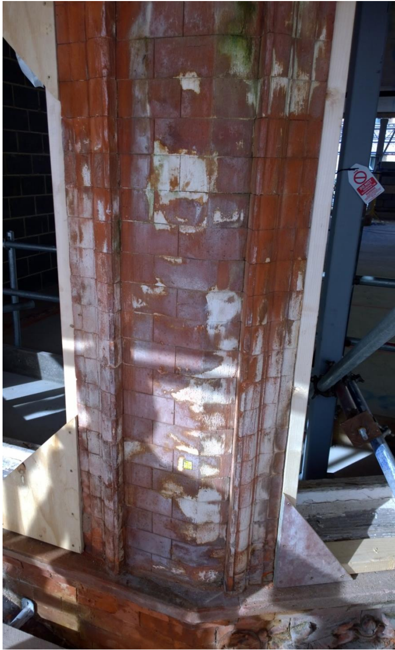
Building no.1 - Retained Façade Failure: Spalling (water ingress)
