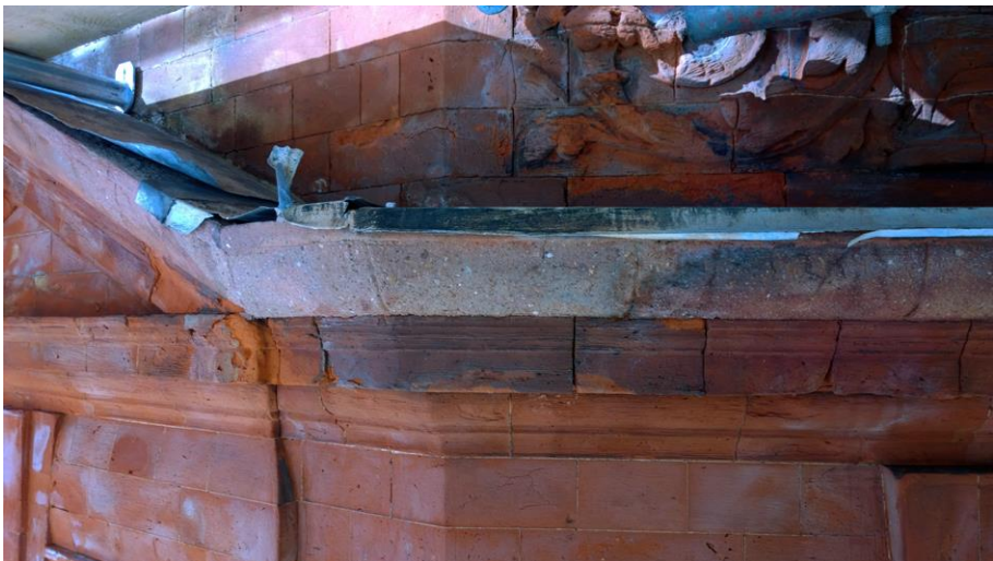
Building no.1 - Retained Façade Failure: Slippage + Movement
