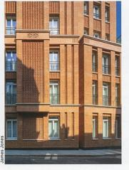
Digital manufacturing and traditional craftsmanship have been combined by the English office Squire and Partners to create a detailed clinker brick facade at Hans Place in London. The office looked into various production methods to produce the decorative bricks and finally opted for a CNC-controlled machine. The bricks were then ground by hand to remove any unevenness in the drill bit. The stones were soaked in water at the construction site before being laid with lime filler.
